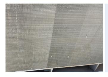
This photo depicts a commercial cooling coil of an HVAC unit on a pier, sitting directly over salt water, running for 3 years.
